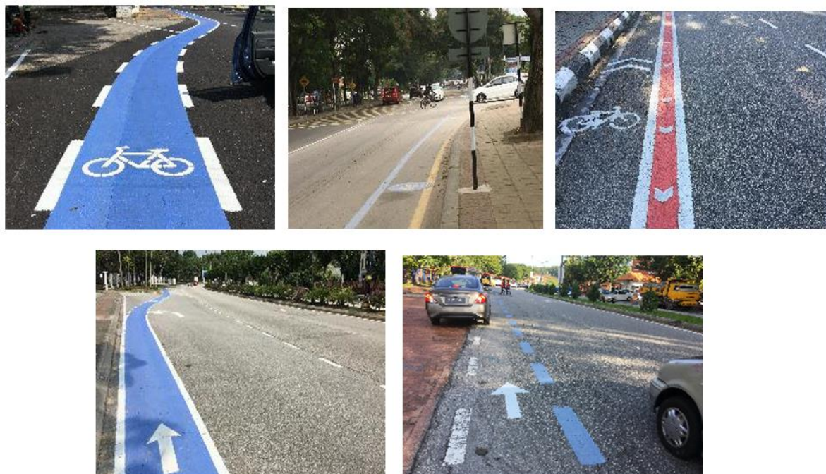
Figure 1: Design of on-street bicycle lanes and signs found during the observation
