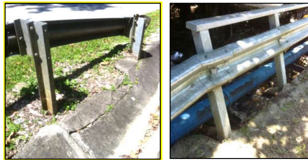
Figure 10: (a) Posts are concreted as < 1000 mm; (b) Pipeline behind the drainage clear zone guardrail with clear zone < 1000 mm
