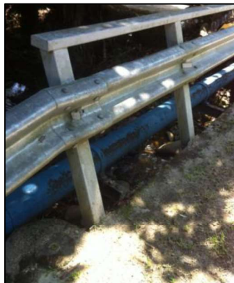
Figure 14: Non-standard posts were used to hold the rail
