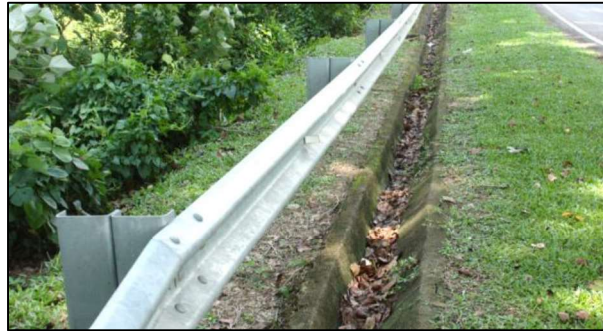
Figure 15: Concrete drain at the front of guardrail installed at rural area
