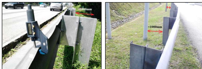
Figure 9: (a) Clear zone > 1000 mm; (b) Clear zone < 1000 mm
