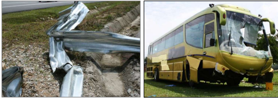
Figure 3: Case study 3 – A guardrail collapsed and failed to redirect the bus
