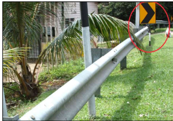
Figure 16: Signage is placed in front of guardrail
