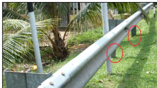
Figure 5: Fixed object is placed less than 1.0m behind pole without concrete
