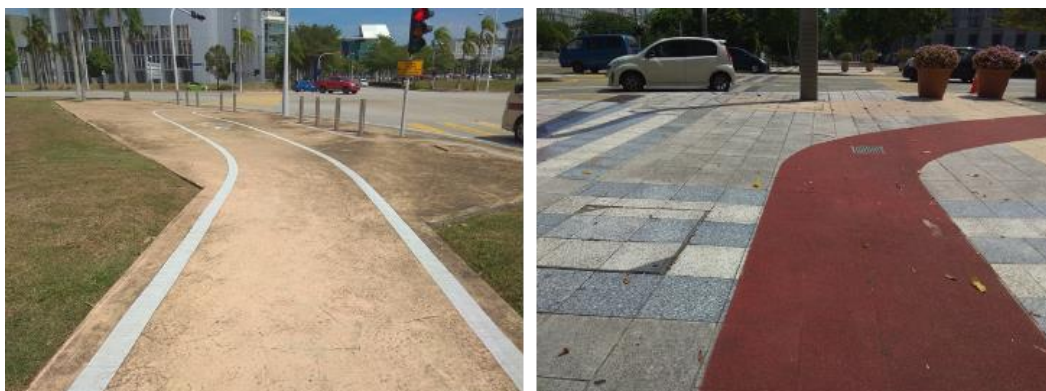
Figure 6: Bicycle lane surfaces in Putrajaya
