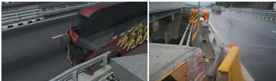
FIGURE 17: The bridge railing penetrated the bus passenger compartment
