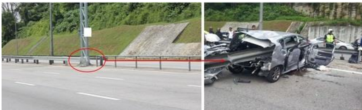
FIGURE 16: The protruding end of the guardrail penetrated the car
