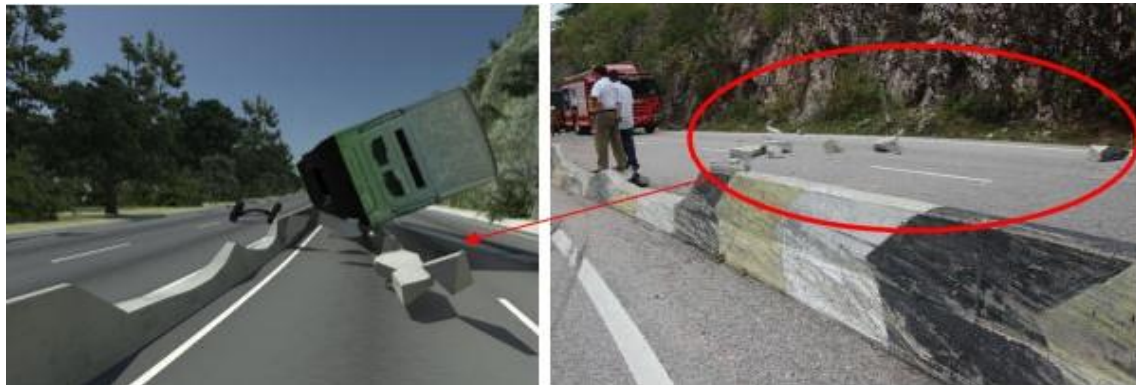
FIGURE 18: The barrier was broken into pieces from the impact and failed to stop the bus from launching into the opposite lane
